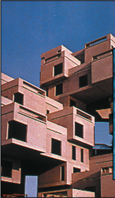
Circa 1967: The Habitat House by architect Moshe Safdie was designed for the year-long Expo 67 in Montreal, Canada. The Housing complex comprised of three clusters of apartments arranged in irregularly stacked blocks.
